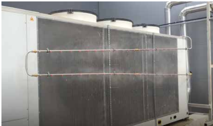
Fig. 1.e - Detail of a chillBooster system installed on a fluid cooler
