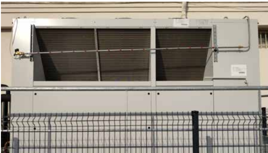
Fig. 1.d - Detail of a chillBooster system installed on a fluid cooler
