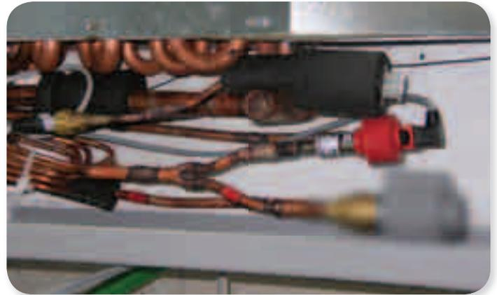
*parallel installation of the E<sup>2</sup>V and PWM valves*
