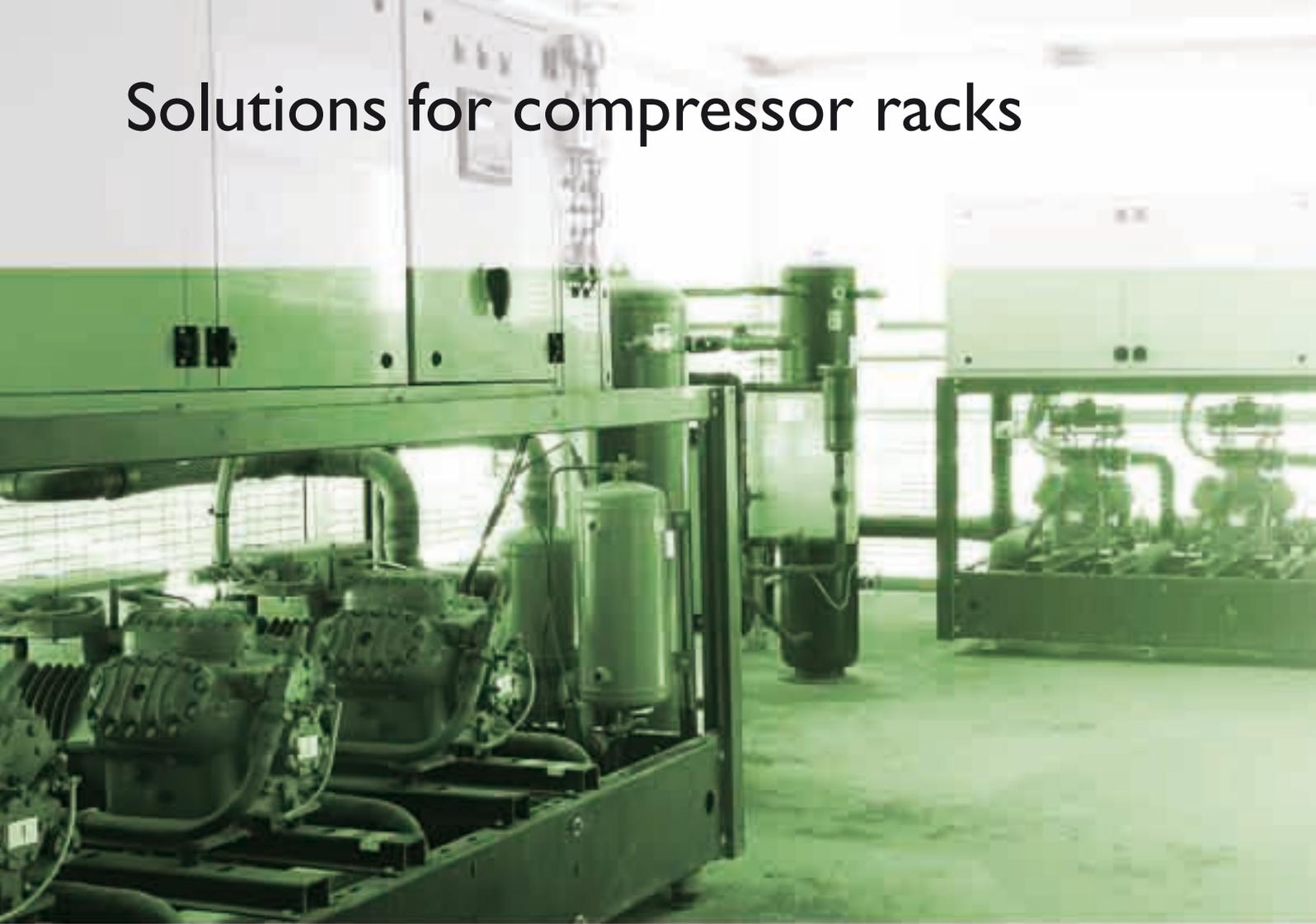
The compressor rack is the most important and complex electromechanical device in the refrigeration system: this delivers cooling for the foodstuffs to all the refrigeration utilities and the related processing rooms.
