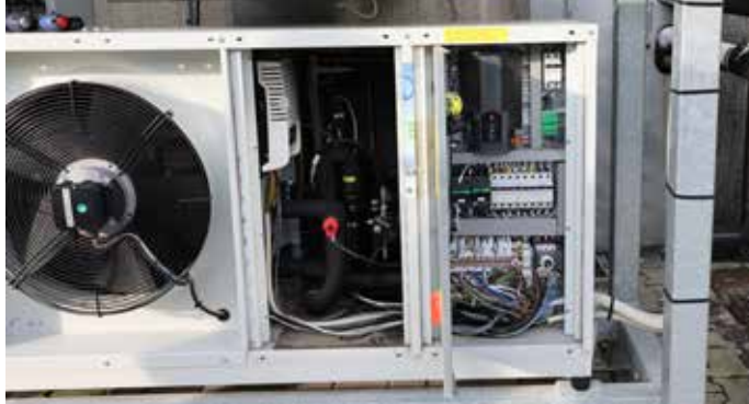
Fig. 1.b - Hecu and PSD2 inverter mounted on the external rack
