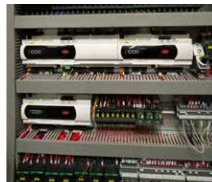
Fig. 1.b - pCO5+ and customised application
