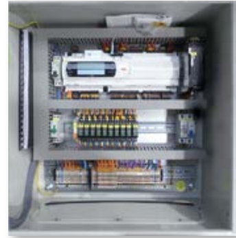
Fig. 1.a - Electrical panels with CAREL electronics
