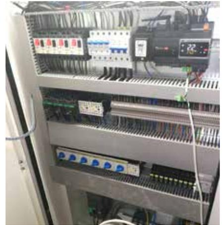
Fig. 1.b -  $\mu$ Rack controller mounted inside the compressor rack electrical panel
