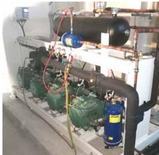
Fig. 1.a - MB Frigo compressor rack equipped with the new CAREL  $\mu$ Rack controller
