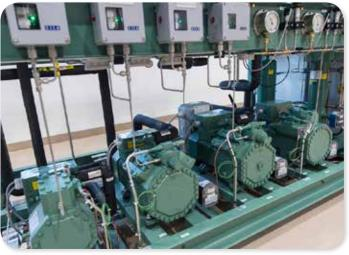
Bitzer compressors for low, medium and intermediate temperature
