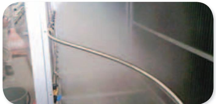
evaporative cooling with atomised water
